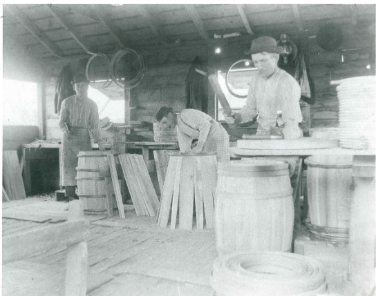
Barrel making at cooper shop, Lockport NY c. 1900
